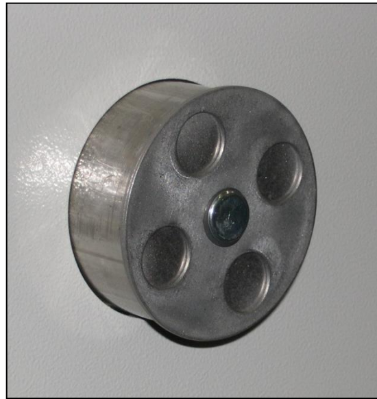
Figure 12. Adjust Damper to Set Exhaust Vent by rotating the outer component.
